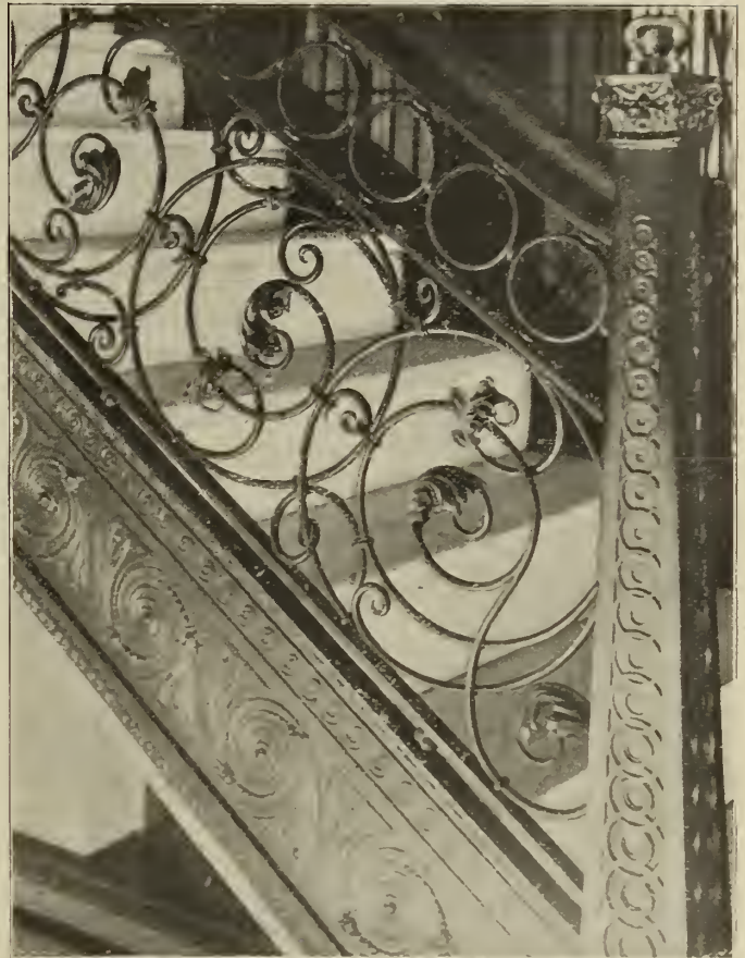
B.—STAIR RAILING, OLD COLONY BUILDING, CHICAGO. Wrought Iron, Hammered Leaf Work, Stringer and Newels Bronze Electroplate.
